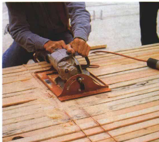
One method for gang-cutting birds' mouths is to cut the heels with a worm-drive saw (photo left) and the seats with a worm-drive saw fitted with a swing table, an accessory base that adjusts from -5° to 68° (photo right). By equipping a saw with a universal dado kit (photo above), birds' mouths up to 3/4 in. wide can be plowed out in a single pass.
